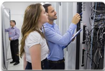
Installations must be inspected for damage.
